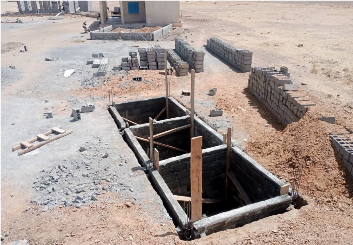
Laying of the bricks completed
