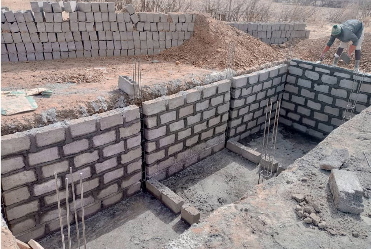
perimeter walls under construction
