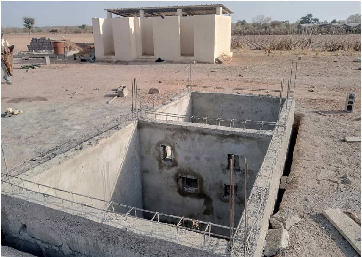
Perimeter walls ready
