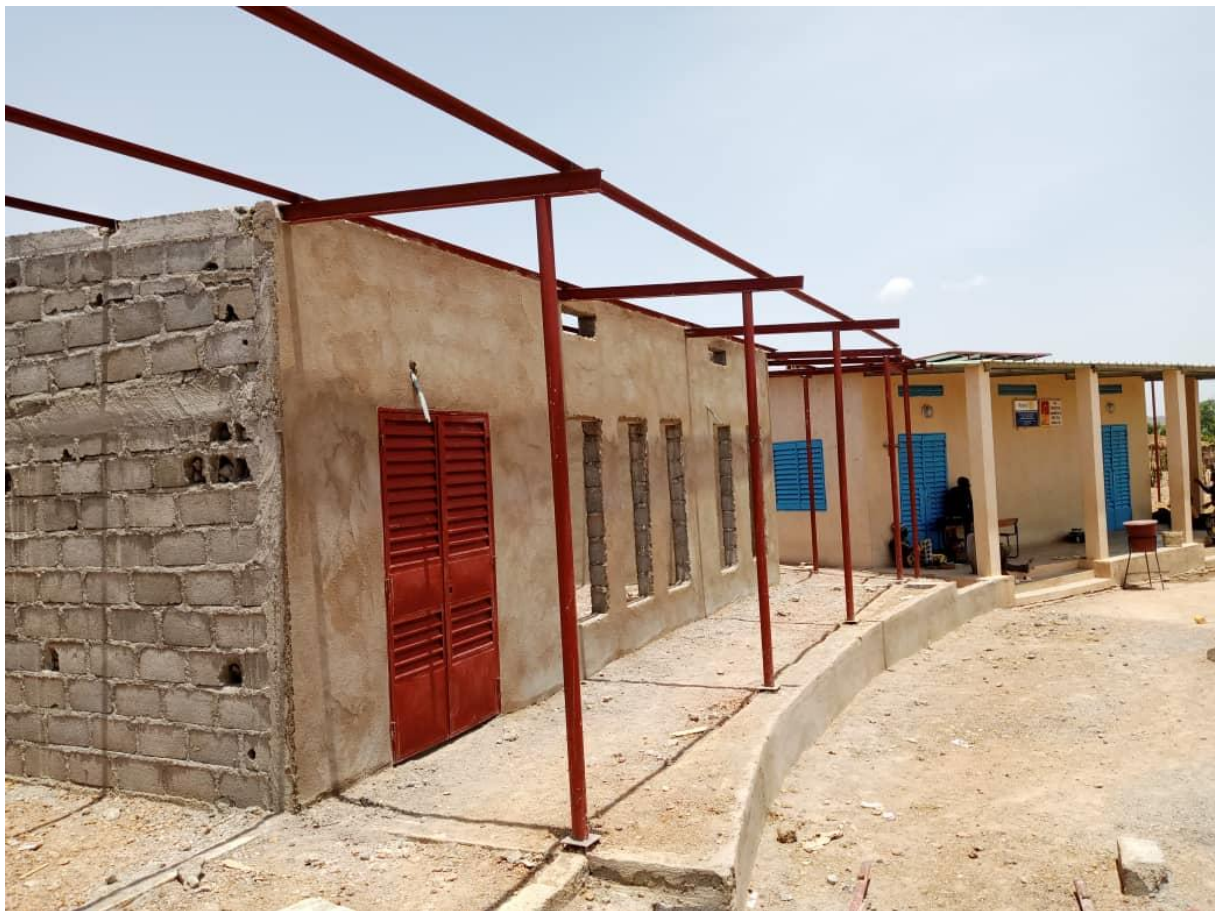
Façade plastering works
