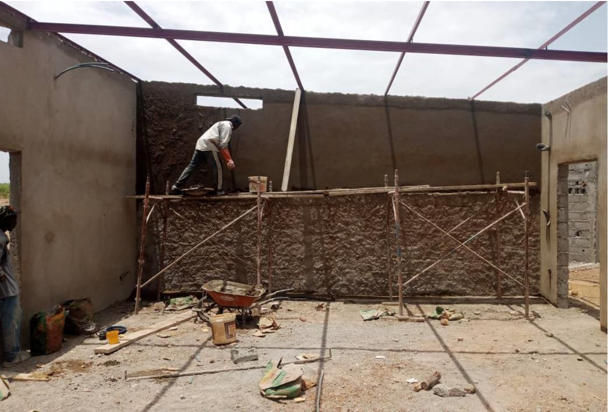
Inside plastering works
