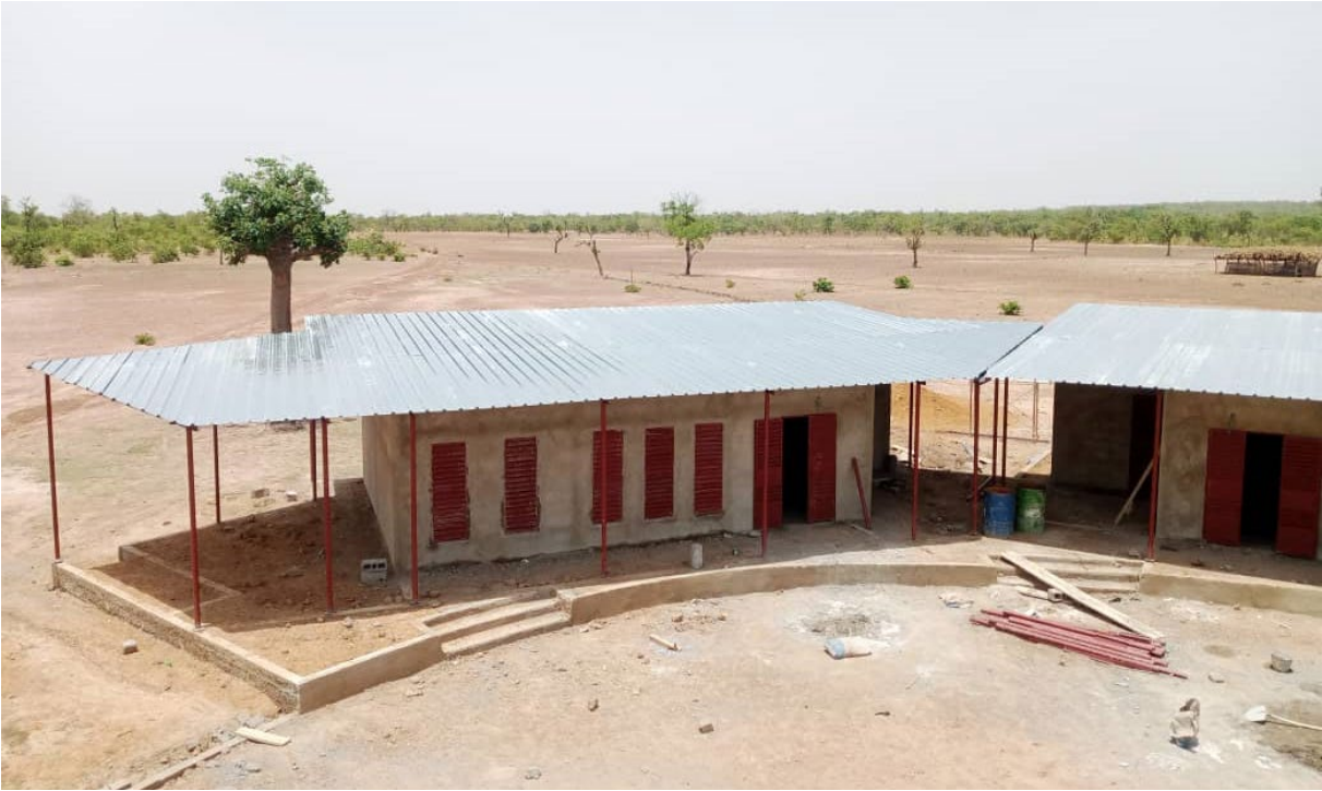
Classroom, roofing, and pedestal.
