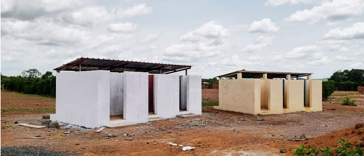
school latrines, second block
