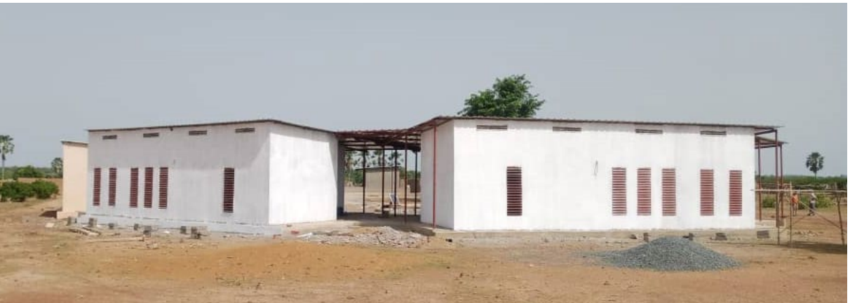
second and third classrooms, back view
