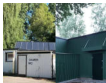
The New Changing Rooms At Rosta Were Ready
